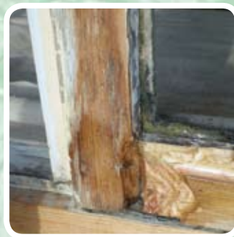
Stabilise sound timber with DRY FIX®.
