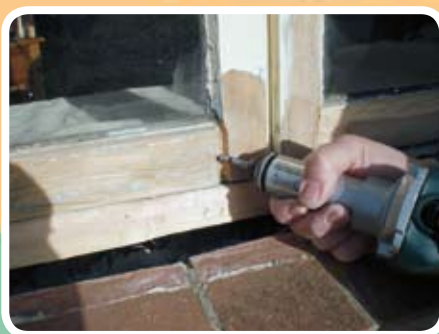
Seal construction joints, splits and shakes with DRY FLEX® resin
