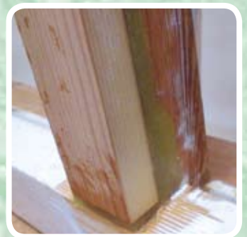
Repair using DRY FLEX® resin or resin and timber.
