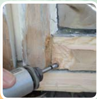
Remove all decay using the Repair Care Mini-PROFI™.
