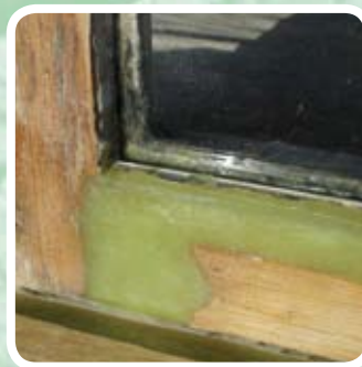
Repair using DRY FLEX® resin or resin and timber.
