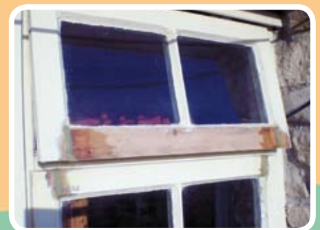
Seal construction joints, splits and shakes with DRY FLEX® resin
